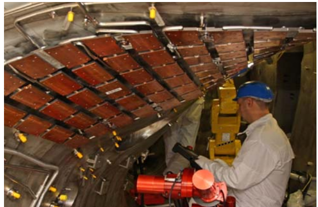
Fig. 2. Heat shields at higher loaded parts of the wall (local design heat load 500 \text{ kW/m}^2 , average load 250 \text{ kW/m}^2 ) during installation in the plasma vessel of W7-X. The water-cooled CuCrZr heat sinks of the shown heat shield segment are not yet covered by their graphite tiles. Photo: IPP, Torsten Bräuer
