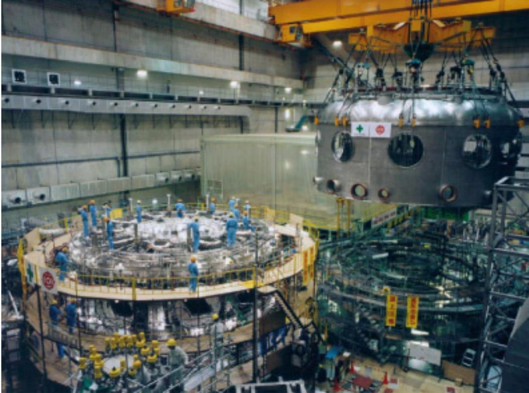
Fig. 3. Moving of the cryostat vessel to the final position.
