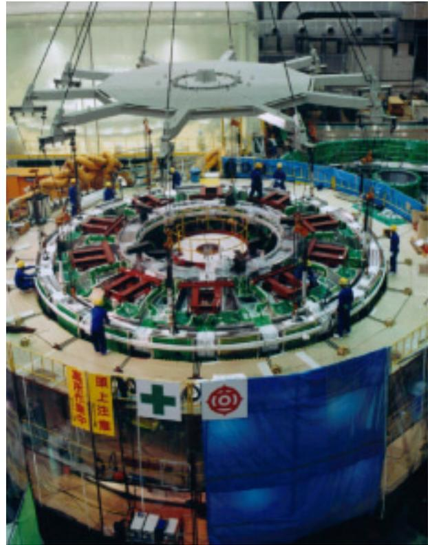
Fig. 2. Installation of the upper outer vertical coil.
